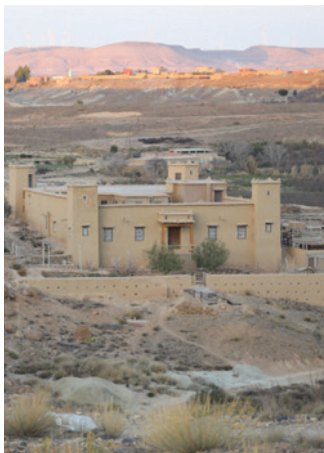
A rural tourist reception structure built using funds provided by returning migrants in Outat valley, Haute Moulouya-Haut Atlas Oriental, Midelt province, Morocco (photo: F. Boukrich).
